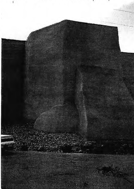
Back Exterior with Buttress
